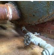
2. Once the buried portion of the tank was cut and hauled away, bricks were carefully removed from the back wall of the pump house to expose the interior of the tank. Finally, the interior portion of the tank was removed. (Note all the rust and sludge inside the tank; the tank was literally rusting from the inside out.)
